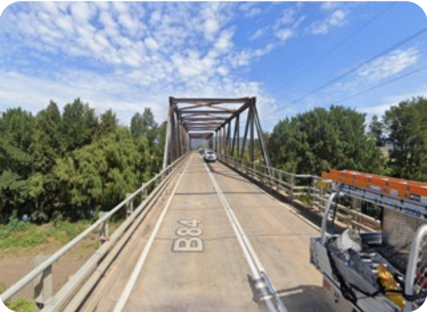
Above: Denman Rd Bridge along Golden Hwy (listed at 5.71m clearance height)
