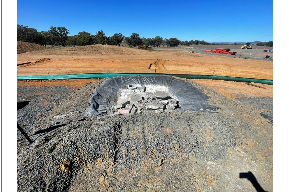
Photo 17 | Transgrid site, dedicated concrete washout bunds with sediment fence behind.
