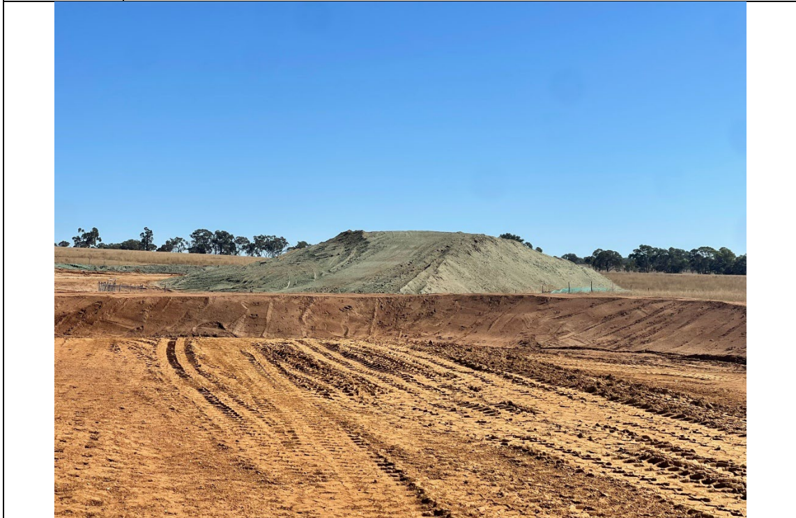
Photo 9 Samsung BESS site, showing soil stockpile sprayed with hydroseed for stabilisation.
