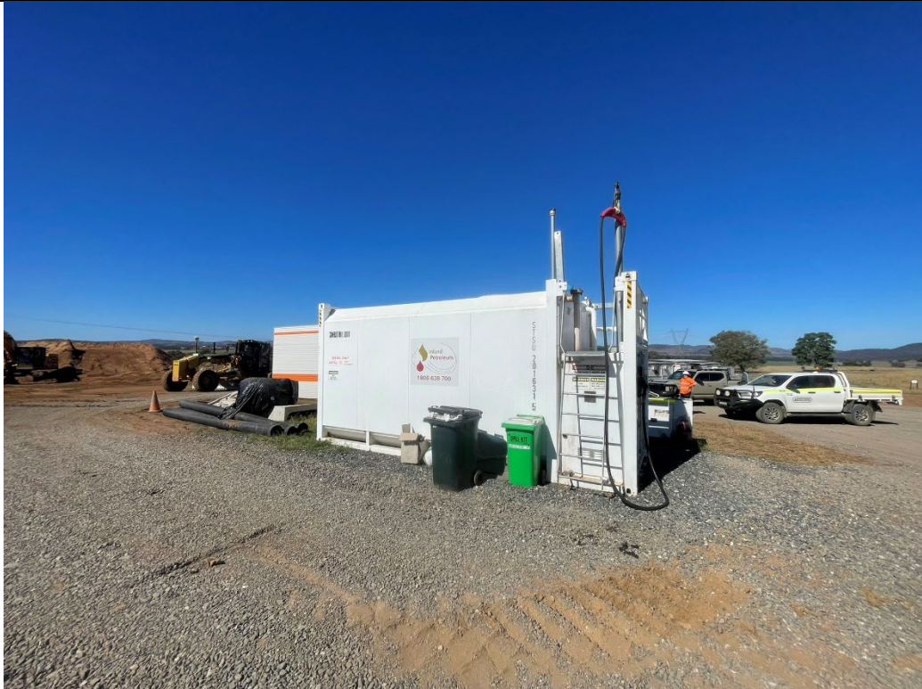
Photo 10 Samsung BESS work site, diesel AST for vehicle refuelling.
