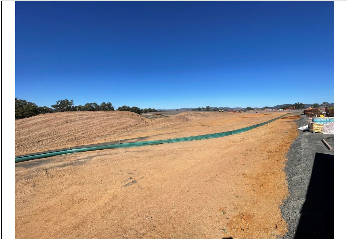
Photo 16 | Transgrid site, showing use of sediment fencing as per the ECP.
