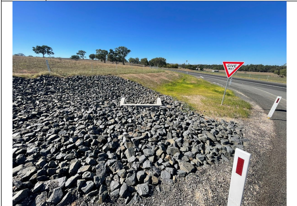
Photo 3 | Recently completed road upgrade works.
