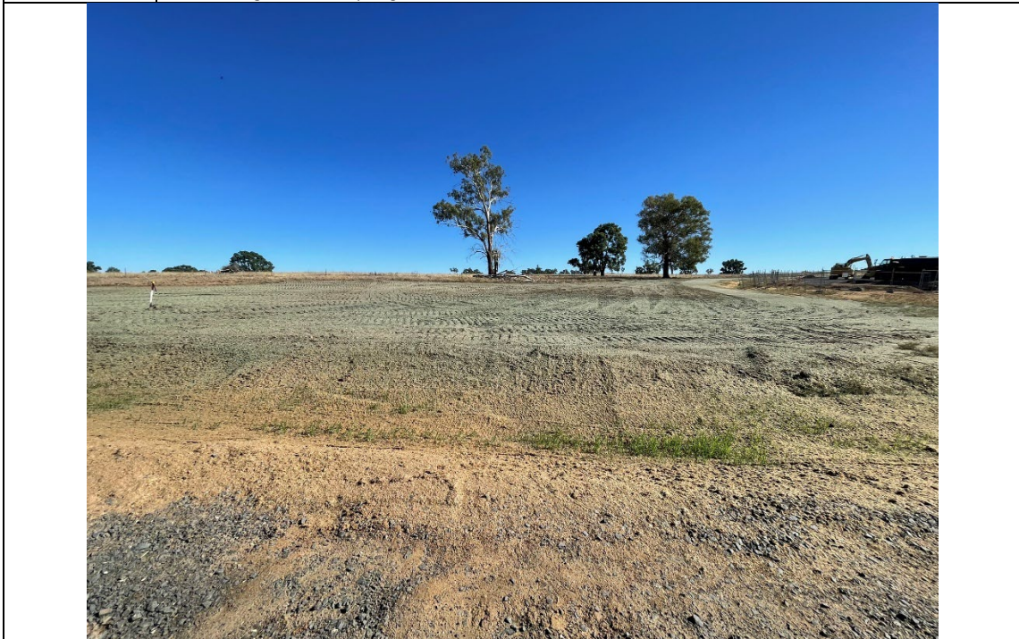
Photo 19 | Previously disturbed area recently hydroseeded as part of rehabilitation.
