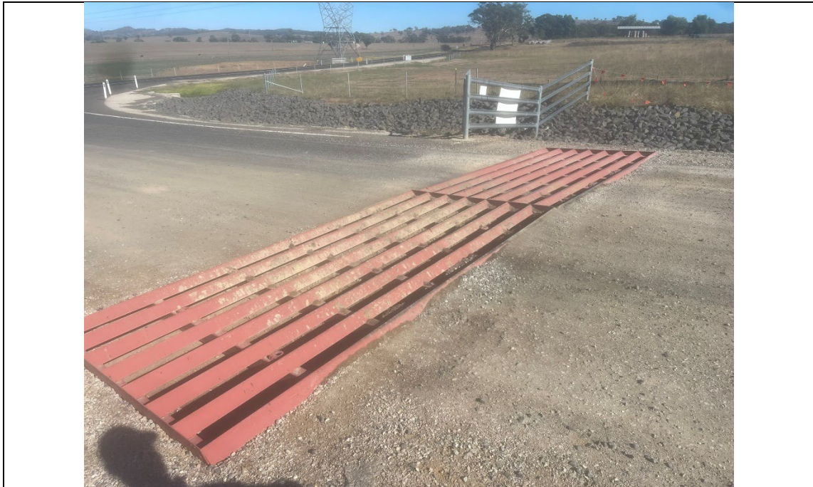
Photo 2 | Main site entrance on Castlereagh Highway, with rumble grid, free of sediment tracking.
