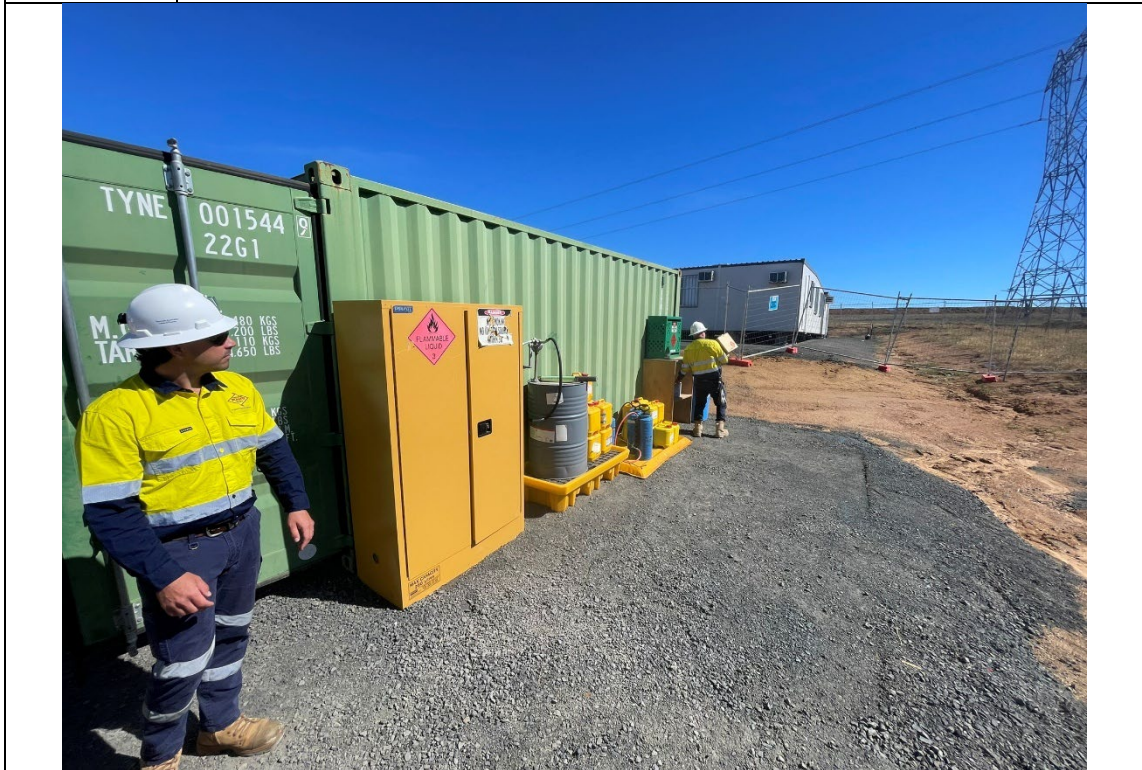
Photo 15 | Transgrid compound, hazardous chemical storage cabinets and oil drums and containers stored on drip trays.
