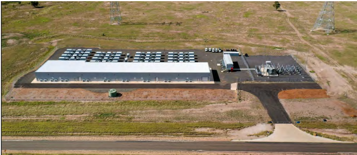
Figure 4-3: Wandoan South BESS, a 100MW/150MWh BESS facility in Queensland, including project substation
