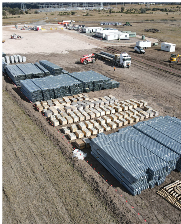
Construction facilities & Laydown area (2022).
